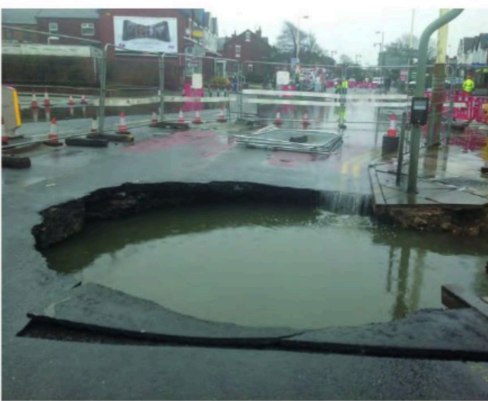
↑ Figure 13.13 Collapsed sewer in Southport.
